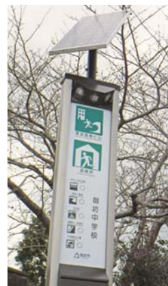
▲既存照明に看板を設置
